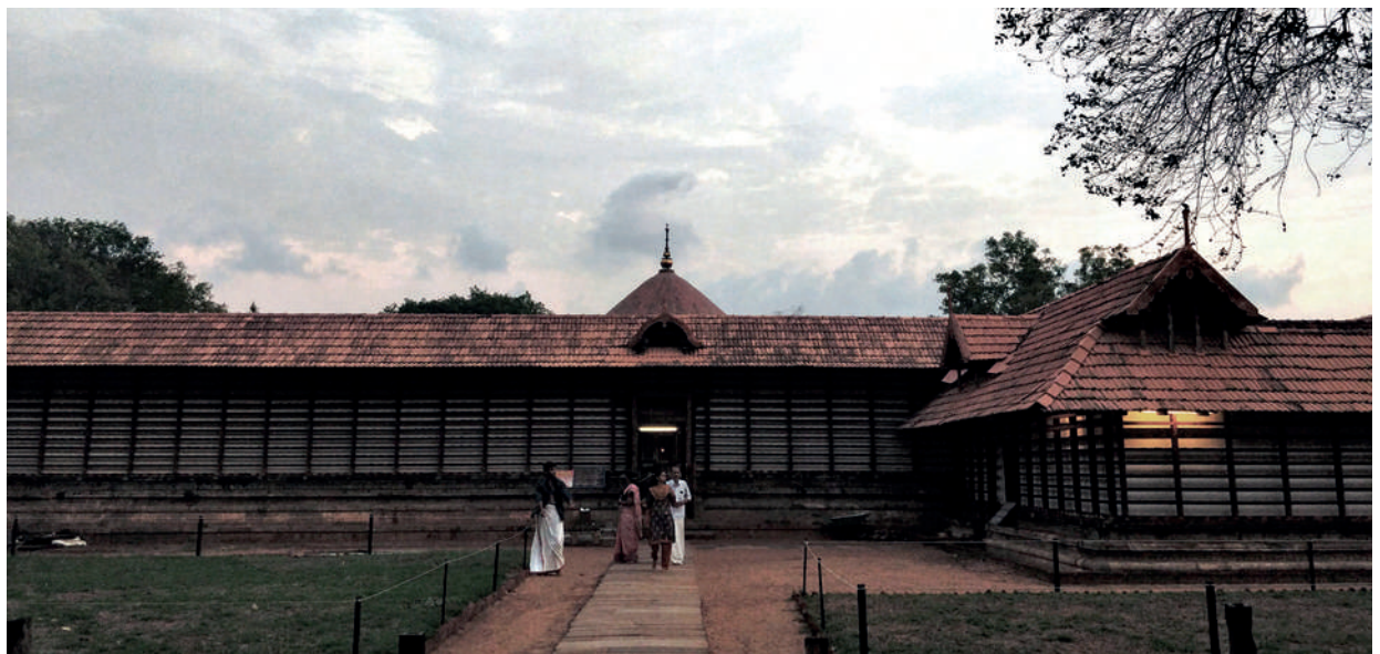
Below: Devotees in traditional outfits exiting the inner sanctum which is enveloped by the corridors and courtyard
